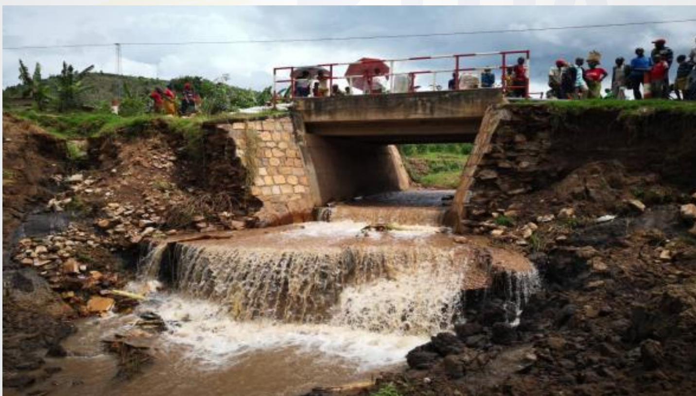
Karama bridge-Wing -walls
