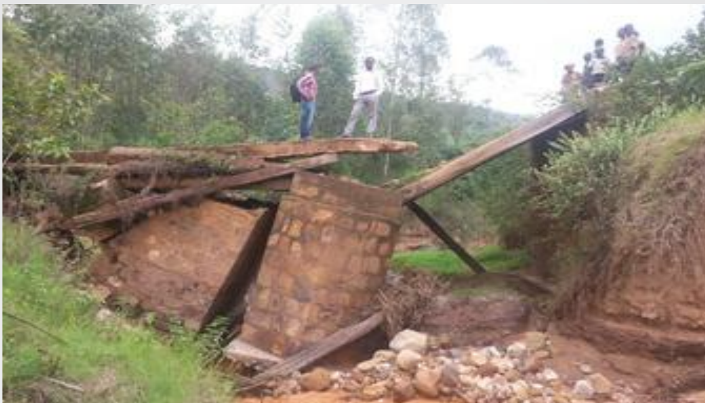
Murambi-Gatwa-Bubangu Road-Wooden bridge
